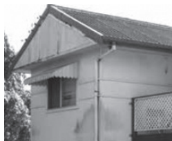
Asbestos Wall Sheeting
