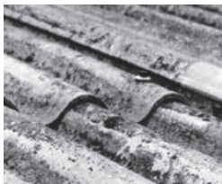
Super Six Asbestos Roof
